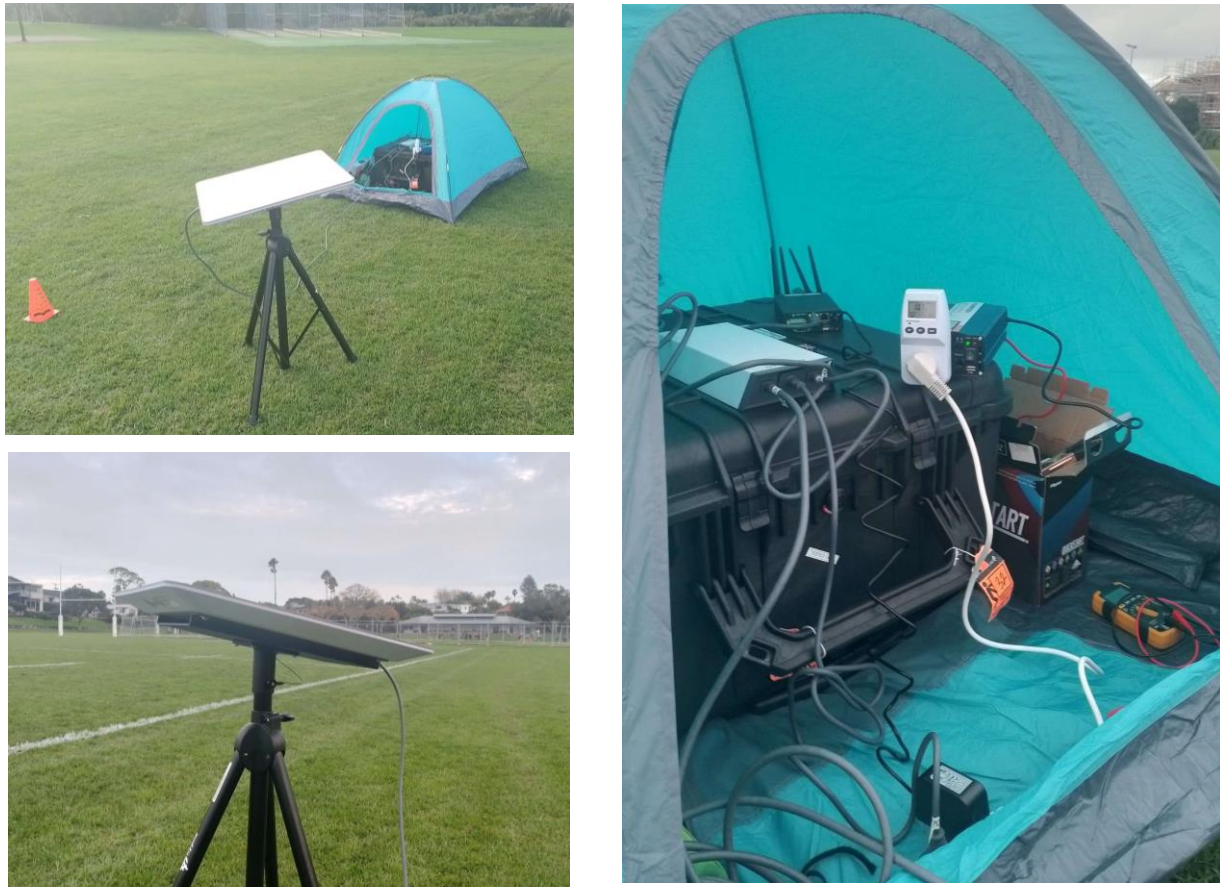
Figure 10: Set-up for Test 9, with battery/inverter as power supply
