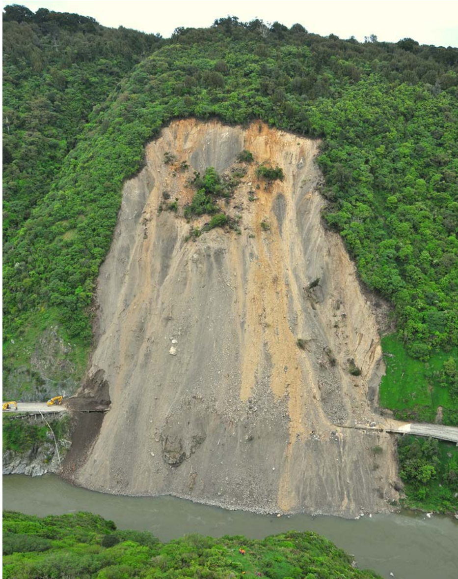
Figure 4.5 A landslide failure during 2011 in the Manawatū Gorge, displaying a cone-like deposit shape (Source: GT Hancox).
